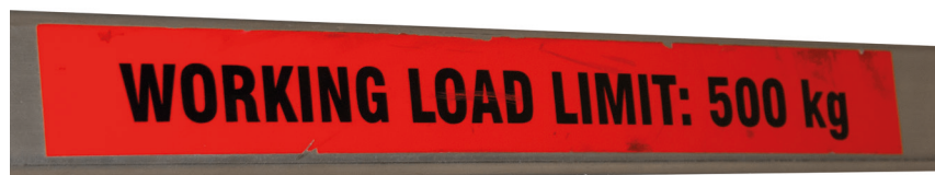
Figure 5: WLL of 500 kg.
