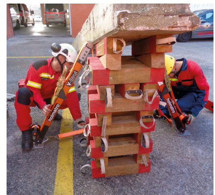
Figure 44: (a) Example of wedges on top of box cribbing. (b) Supporting a slanting load with box cribbing and wedges.
