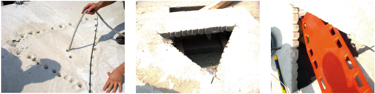
Figure 40: (a) Triangular clean breach being prepared. (b) Final result of the clean breach. (c) Spinal board being passed through the breaching.
