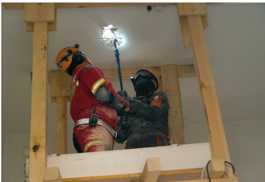
Figure 35: Vertical class 3 shoring with integrated working platform.
