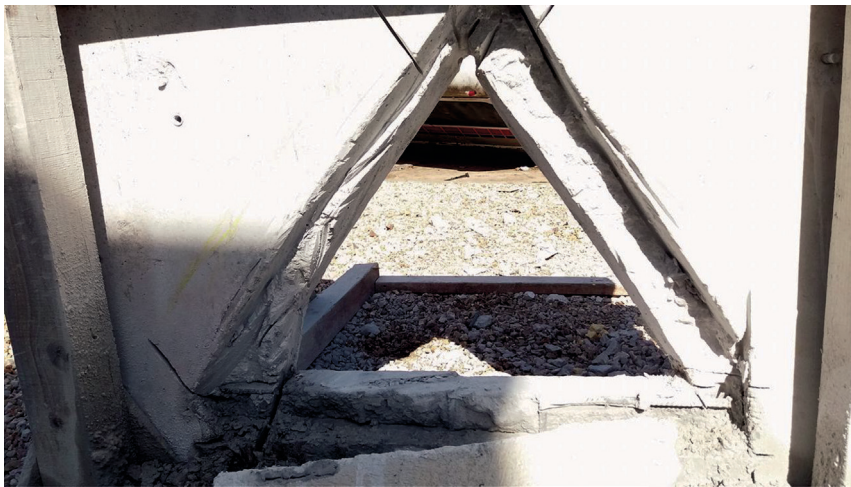
Figure 41: Final result of a step cut in a concrete wall.
