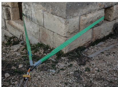
Figure 39: Anchor mounted on a built structure.
